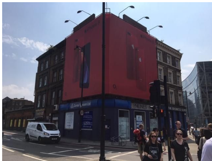
Fig 3. 32 Shoreditch High Street
