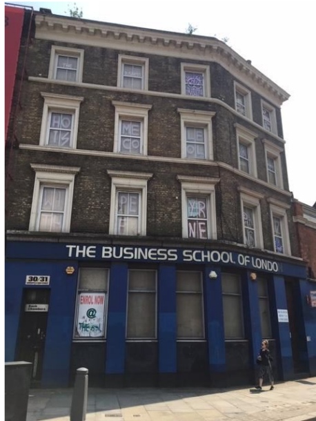
Fig 2. 27 – 31 Shoreditch High Street
